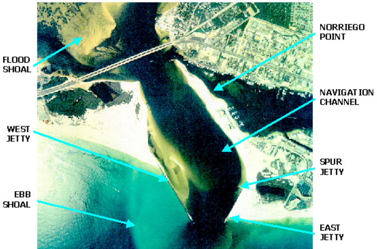
Figure 7. East Pass, Florida, U.S.A. Aerial photo taken in 1989. North is to the top.
